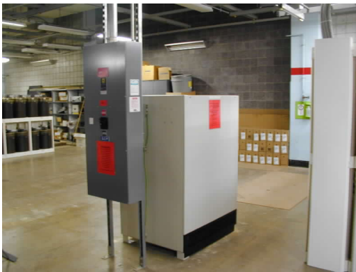
Figures 1 and 2. Cabinetized VRLA batteries share a spacious power room in this UPS application.
