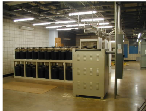
Figures 1 and 2. Cabinetized VRLA batteries share a spacious power room in this UPS application.
