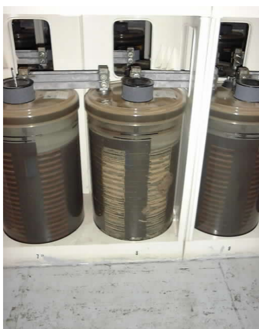
Figures 7 and 8. Severe cell sulphation.
