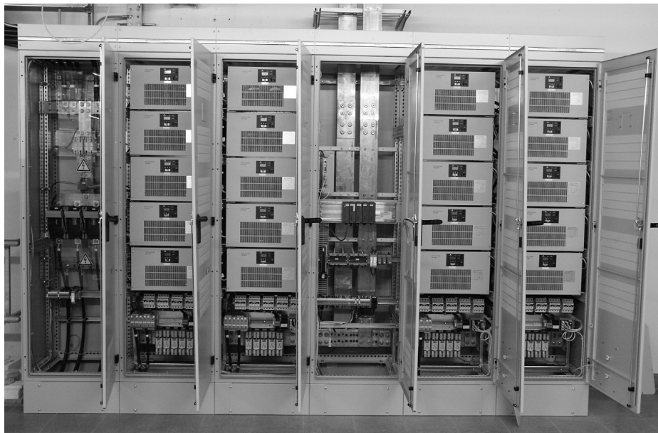
Figure 5: 285VDC/60VDC DC/DC Converters 290kW
