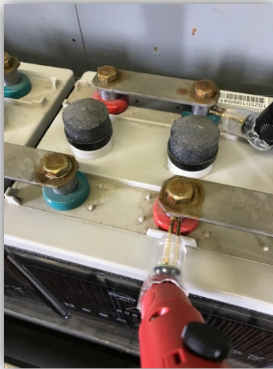
Figure 2. A cell conductance (internal ohmic) test
