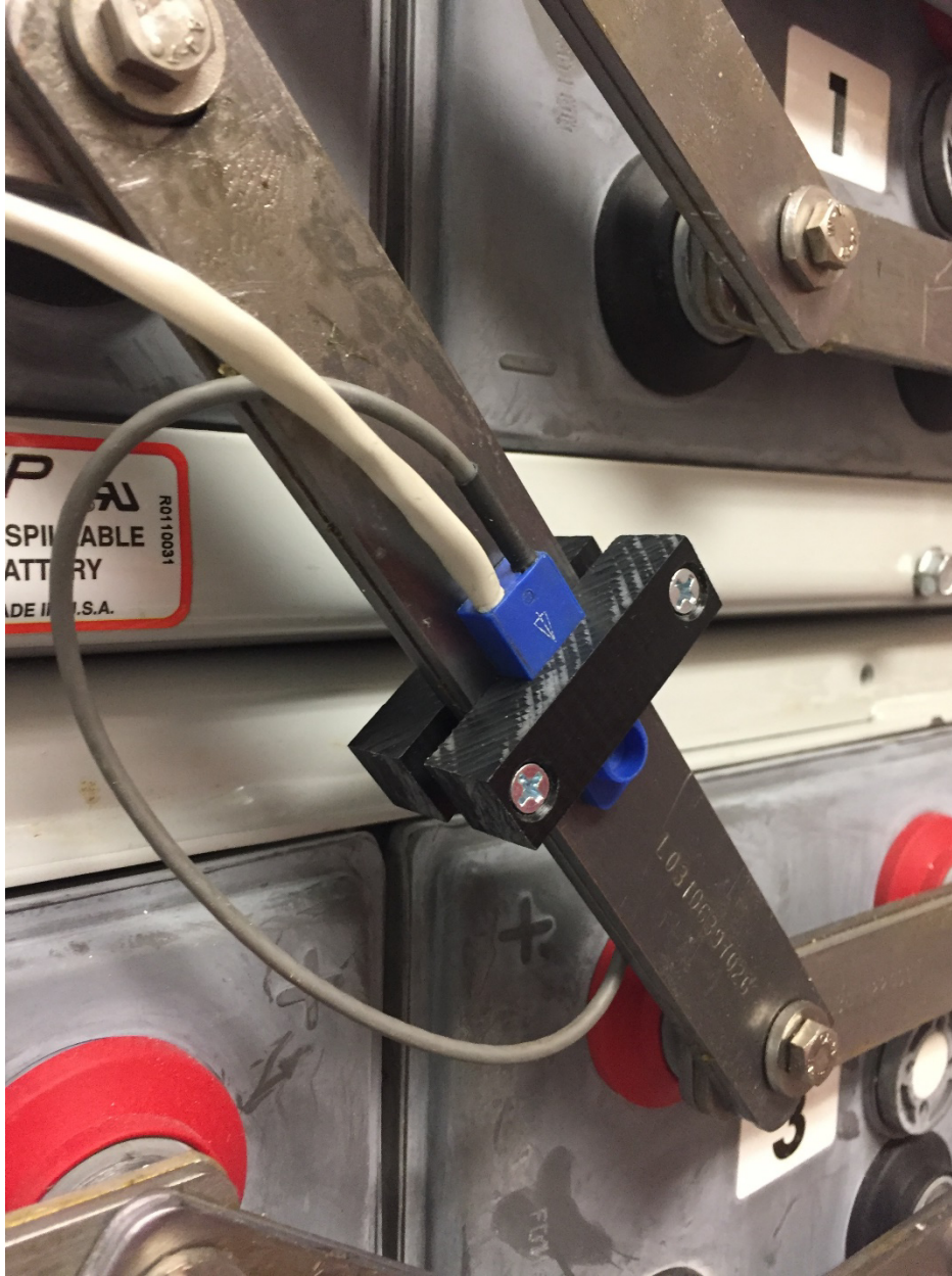
Figure 8. Current sensing part of a BEM (Battery Event Monitor) unit, which also monitors the OAV (overall voltage), cell temp, and ambient temp, and has adjustable alarm thresholds for each value, and can be installed without interrupting the circuit.
