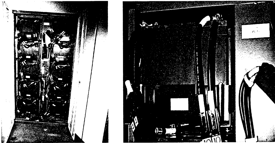
Typical UPS battery cabinet with 12 volt modules. There is practically no access to the terminal posts.
